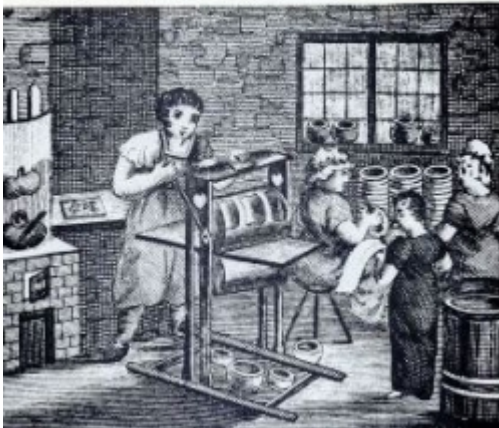
Printing on thin paper, impressions transferred to the fired ware, and paper washed off.
